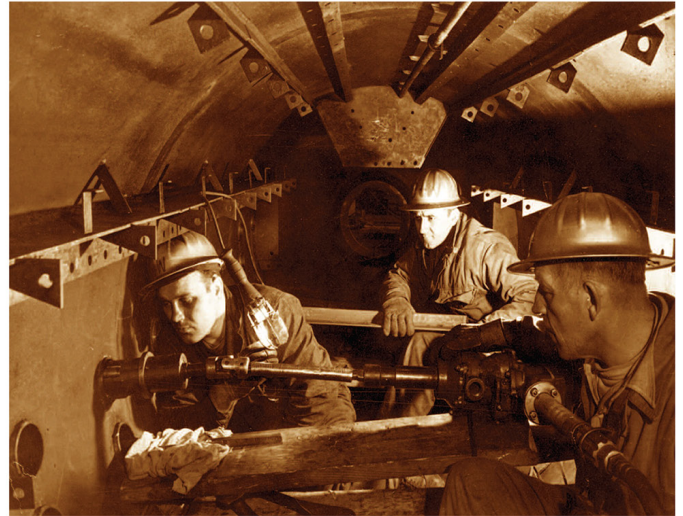
Rolling tubes, Boilermakers at work
