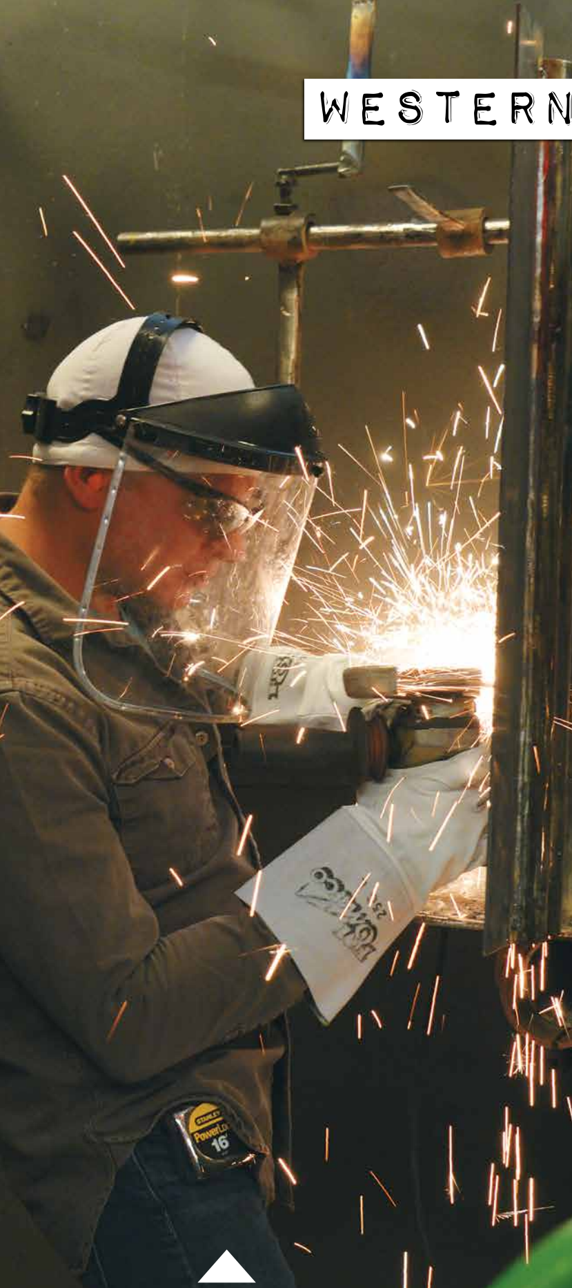
MIRCHA VOROBETS, L-242 , removes a tube from a simulated waterwall panel using an angle grinder with a wafer wheel.
