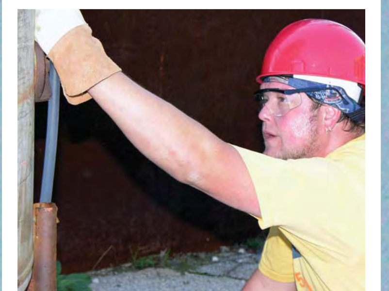
Brian Beach (L-11) uses a water level to level a vessel.
