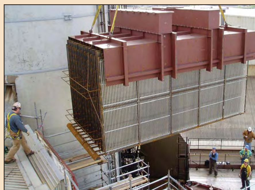
The agglomerator is lifted up so it can be attached to the front of the unit's electrostatic precipitator.
