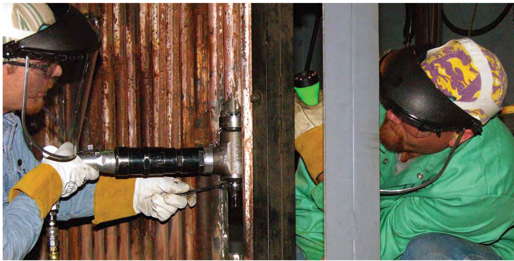
Jimmy Sutton (L-453) and Jeremy Grubb (L-105) work as a team to mill a tube.
